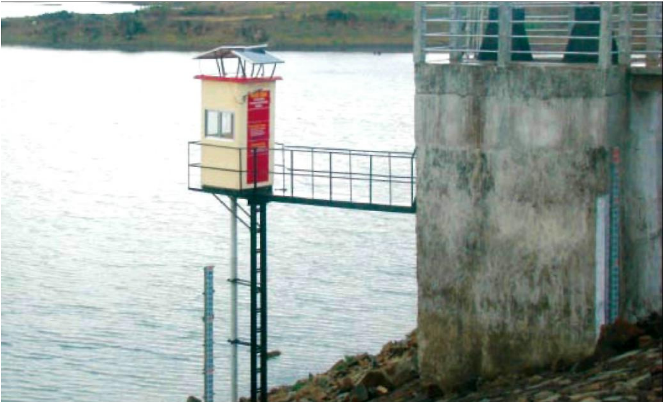
Installation of Automatic Water Level Recorder at Nesa Dam
