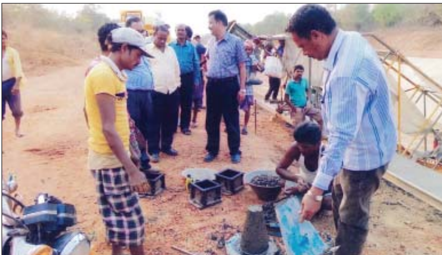
Slump & Cube Testing of CC lining of canal at Subarnarekha Irrigation Project
