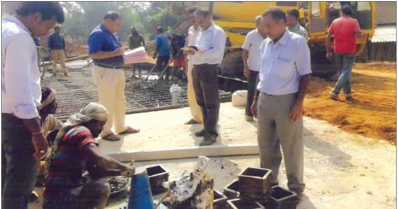
Slump & Cube Testing at Subarnarekha Irrigation Project
